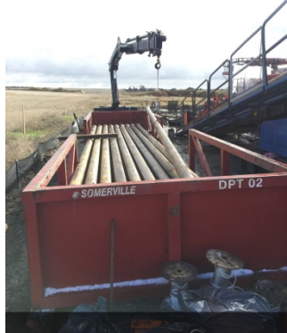
Sept 28/18 Description & Location: SSKP 899+350 HDD Bore site Black Creek This is where they store rods for bore They use hoist for hooking up and dismantling rods, facing east
