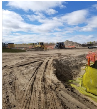
Sept 28/18 Description & Location KP-826 + 745 Photo taken facing west. Worker spraying down his truck. Dozer parked
