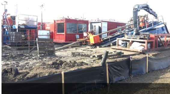
Sept 28/18 Description & Location: SSKP 899+350 HDD Bore site Black Creek Currently reaming with 42" bit Operator in dog house with windows - Facing SW
