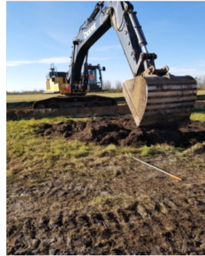
Sept 25/18 Description & Location: KP 811 + 300 Photo taken facing south. Excavator removed the contaminated soil, than replaced it with fresh top soil at SF # 28
