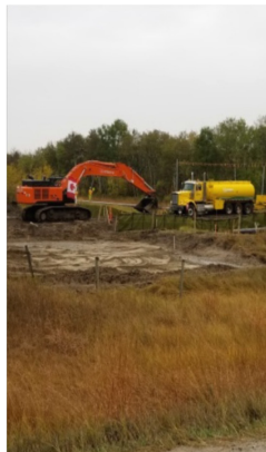
Sept 26/18 Description & Location: 819+432.5 148 west Photo taken facing south Excavator pulling tank truck from SF # 13 to SF # 12
