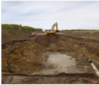
Sept 25/18 Description & Location: KP 830 + 899 Photo taken facing west Excavator digging the open ditch ay SF # 23
