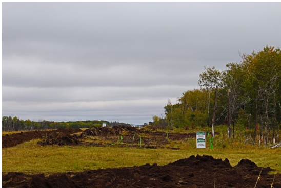
Sept 24/18 Description & Location: SSKP 855+115 Broad-Leaf Treed Swamp Wetland MB-081 Grade crew has started to strip by wetland This area wasn't bad for rain Facing East
