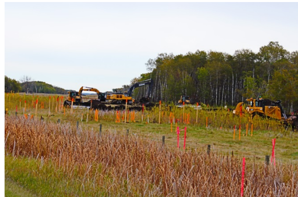
Sept 25/18 Description & Location: SSKP 835+735 Grade Crew stripping around wetlands Dozers and Excavators Stripping soil Lots of buried facility's mostly MTS Facing south east
