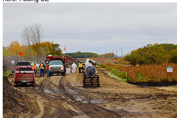
Sept 24/18 Description & Location: SSKP 817+665 Coating off sections at Rd # 6 Blasting pipe on left side Coater in white waiting to paint – Facing West
