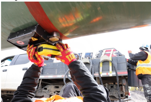
Sept 27/18 Description & Location: SSKP 812+700 Isolated Induction Coil for repairs This device is much more safe for repairs Worker heating repair at 6'o clock, Device in hands on pipe
