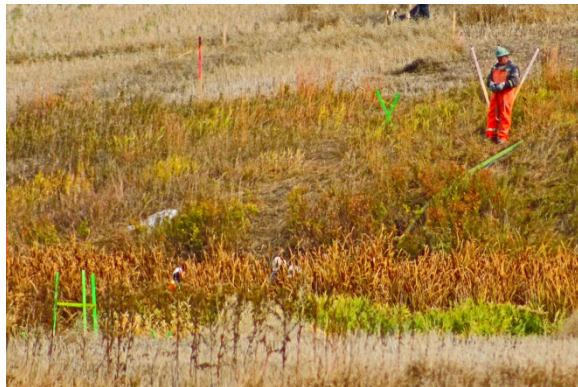
Sept 25/18 Description & Location: SSKP 899+760 Frack fluid coming through surface in Black Creek, Environmental Inspector at left Badger worker middle using suction & water Operator to right, facing east
