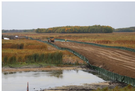
Sept 26/18 Description & Location: SSKP 848+ 750 Semi-Permanent Marsh Class 4 MB-071 A small pond south of wetland ramp Facing north west
