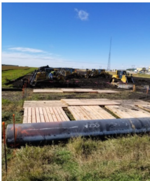
Sept 26/18 Description & Location KP-873+696.2 118 west Photo taken facing west Prepping to build a ramp under the road way
