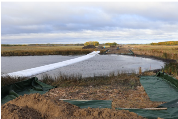
Sept 27/18 Description & Location: SSKP 848+400 Aqua Dam just completed Draining water to left of dam If you zoom in you can see 6 ducks to right Facing west
