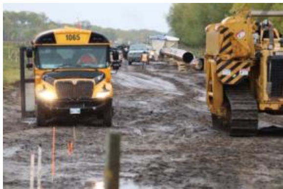
Sept 26/18 Description & Location: SSKP 841+750 Welding a bore section in wetland Bus parked close to crossing as ROW is wet Side Boom waiting to be loaded Facing east
