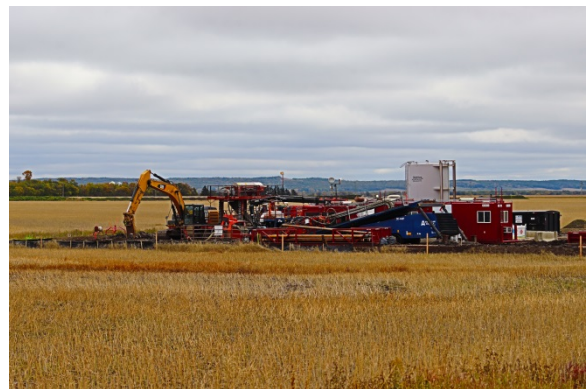
Sept 24/18 Description & Location: SSKP 899+250 Somerville HDD site on Banister ROW Banister is prepping pipe to be pulled Once they weld pull head on bore section they will pull it from here. Facing SE
