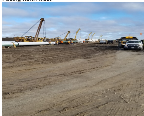
Sept 27/18 Description & Location KP-821-200 Photo taken facing west. Prep gang preping the pipe for the welders Main gang welding the pipe.
