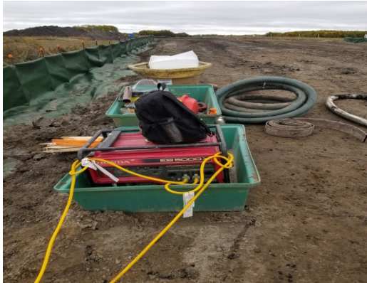
Sept 27/18 Description & Location KP-848+350 Photo taken facing west. Generator and fuel jugs are well contained. At SF # 29 wetlands complex MB 0571. Semi permanent class four.
