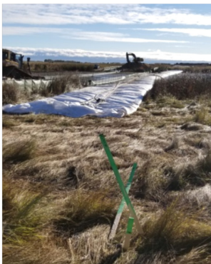
Sept 28/18 Description & Location KP- 848 + 400 Workers putting up the fence Clean and tidy MB 071. Wetlands complex. Class 4
