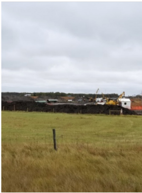
Sept 24/18 Description & Location KP- 821+006.251N Photo taken west. Side booms moving welding shacks. Very congested and muddy
