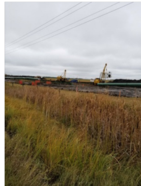
Sept 24/18 Description & Location KP-819+432.5 148 west Photo taken facing east. Pipe gang continuing welding
