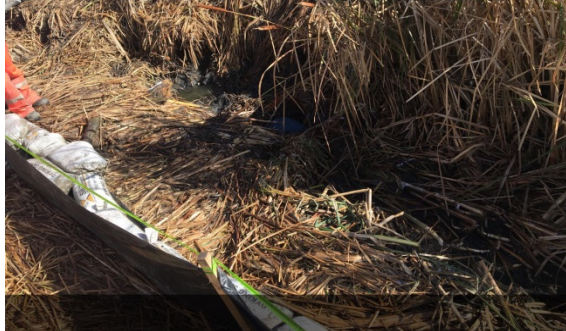
Sept 28/18 Description & Location: SSKP 899+650 Location in Black Creek Frack fluid came through surface here They did a good job containing it Very good work by Enbridge & Badger
