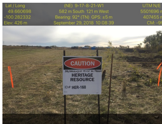
Sept 29/18 Description & Location: SSKP 863+050 Heritage Resource area Only can strip soil with Archeologist present Some already stripped to the right - Facing East
