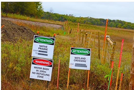
Sept 24/18 Description & Location: SSKP 821+100 Native Prairie and Wetland Work in area is ongoing Bore pipe installed under road- Facing North
