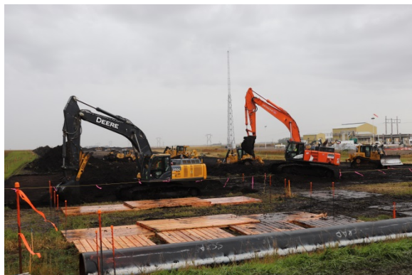
Sept 26/18 Description & Location: SSKP 873+800 Grade crew stripping by road crossing Flume pipe ready for road approach Enbridge Souris Station in upper right Facing north west
