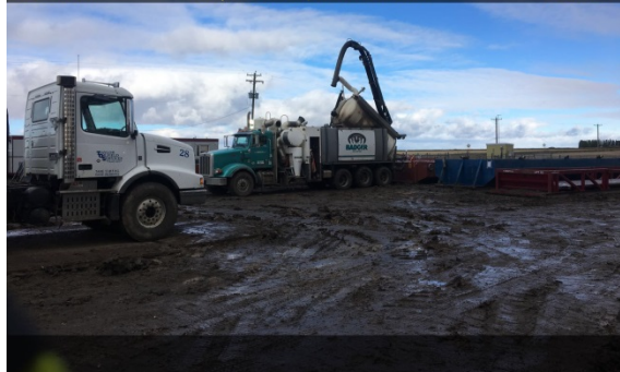
Sept 28/18 Description & Location: SSKP 899+350 HDD Bore site Black Creek Badger hydro-vac dumping bad soil in bin Conditions on site still slippery
