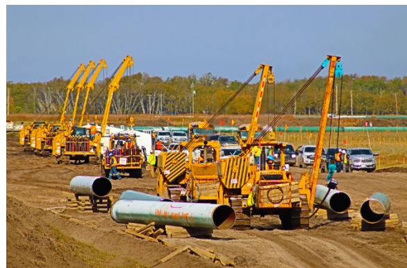
Sept 25/18 Description & Location: SSKP 823+025 Pipe Gang Welders in Wetland MB-1039 Just finishing there welding in wetland Soil condition was starting to dry more Facing west
